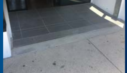
AWMA Concealed Flood Barrier Stage 3 - Conceal
