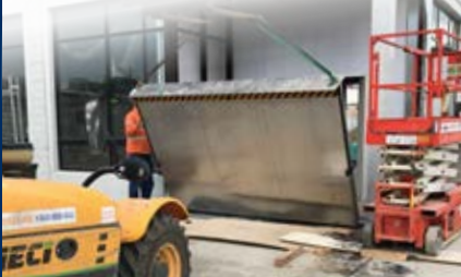
AWMA Concealed Flood Barrier Stage 1 - Construct
